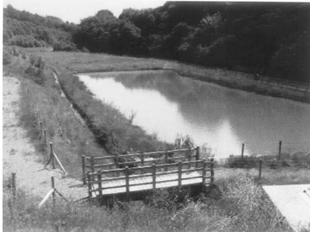
Figure 8.4 Taff Merthyr mine water treatment scheme, South Wales. (a) When Taff Merthyr, Deep Navigation and Trelewis collieries closed in 1990, mine water rebound resulted in discharge from two shafts at Taff Merthyr Colliery causing pollution of a 3 km stretch of the Bargoed Taff, a tributary of the River Taff. The treatment scheme is an aeration and settlement system to facilitate oxidation and settlement of iron. A series of aerobic surface flow reed beds follow the aeration and settlement treatment. There are 16 wetland cells with a fall of 1 m between cells to re-aerate the water by means of cascades. The sludge in the settlement tanks needs to be emptied every five years, the parallel arrangement of the system allowing one tank to continue in operation while the other is emptied. (b) Reed beds following aeration and settlement. (Reproduced by kind permission of the Coal Authority.)
